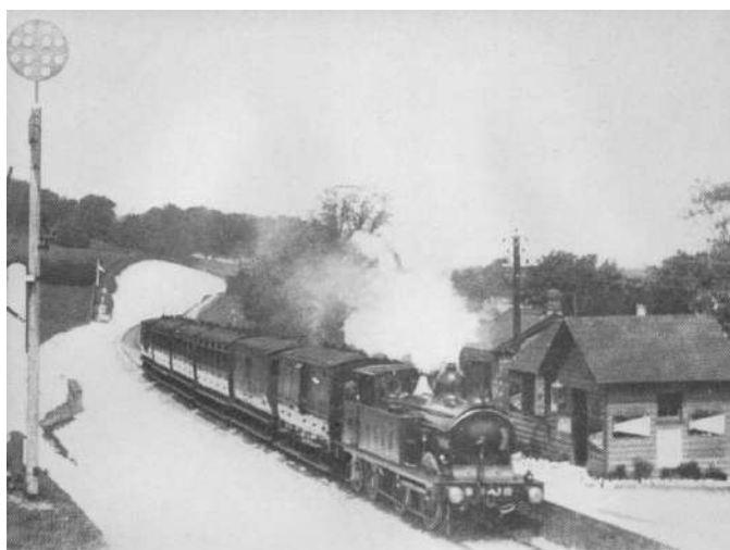
widening work in progress through the chalk circa 1899 as a train arrives from Blandford
