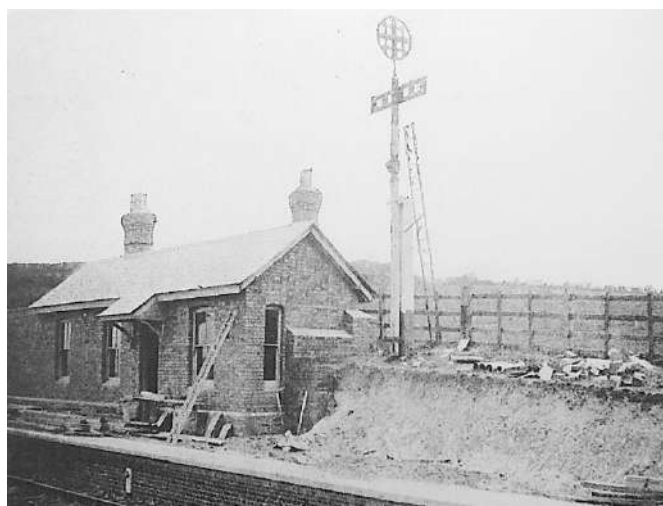
construction of the 'up' platform station building nearing completion circa 1901
